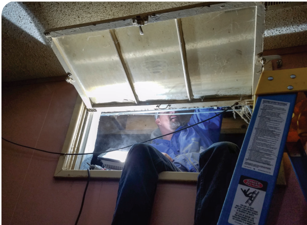
Brent Faurot of Faurot Heating and Cooling works on a new supply line to improve the air flow to a room addition in Cindy's house.
