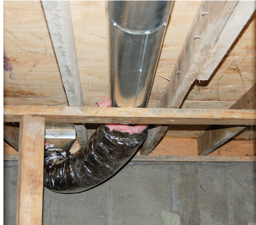
A view of the new supply line that will carry more air volume and to a better location in the room addition.
